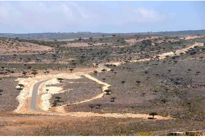
Destruction to vegetation and natural habitats is massive along poorly built roads, such as near Diksam, Oct 07.
